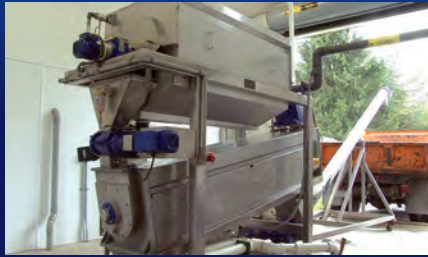
DSP Screw Press Model 3012, NY WWTP
