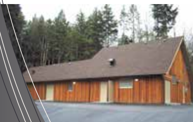
NO NOISE, OUT-OF-SIGHT WWTP
