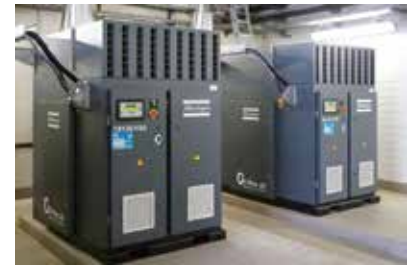
Fig. 3: Atlas Copco ZB Magnetic Bearing /High Speed Turbo
