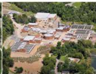
Flavelview Wastewater Treatment Plant, ON
