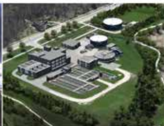
Owen Sound Wastewater Treatment Plant, ON
