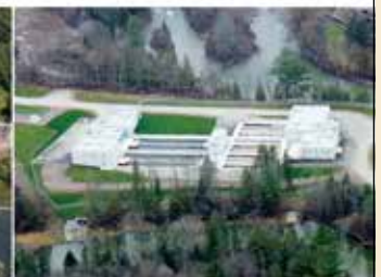
Parliwast Wastewater Treatment Plant, ON
