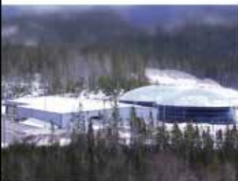
Corner Brook Water Treatment Plant, NL
