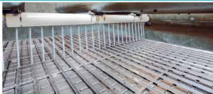
Phoenix Panel System with Air Scour
