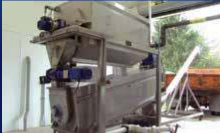
DSP Screw Press Model 3012, NY WWTP
