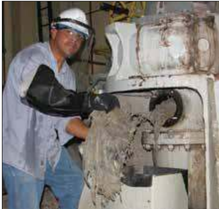
A senior mechanic performs routine dragging in an Orange County Sanitation District lift station pump. Photo courtesy of Ingrid Hellebrand, Orange County Sanitation District.
