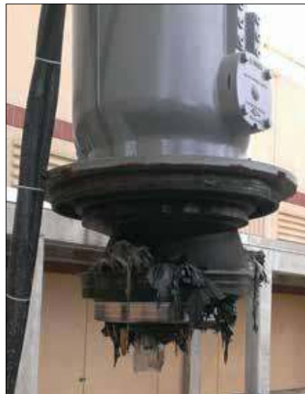
A DC Water (Washington) pump clogged by nondispersible items flushed down the toilet. Photo courtesy of Hiram Tanner, DC Water manager.
