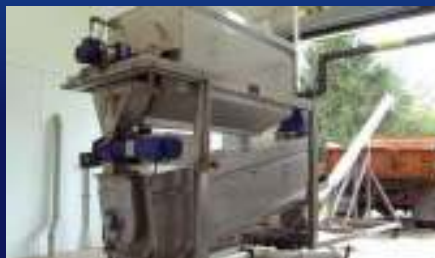
DSP Screw Press Model 3012, NY WWTP
