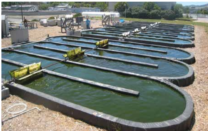
Figure 2. Raceway algae high rate pond Credit: Lundquist, T., Spierling, R., Parker, L., Pittner, C., Medina, L., Steffen, T., Alvarez, J., Adler, N., and Benemann, J. (2016). "The RNEW® Process: Recycled Water, Fertilizer, and Power from Wastewater," presented at Algae Biomass Summit, Oct. 23, 2016, Phoenix, Ariz.
